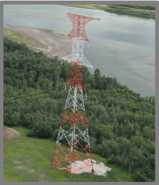
138kV Double-Circuit Lattice Tower Structure
