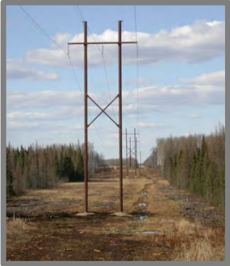
138kV Single-Circuit H-Frame Structure
