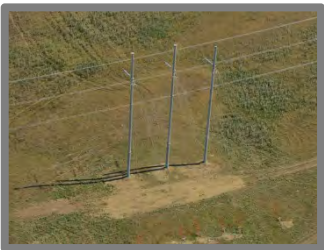
Guy-Anchored Tap Structure
