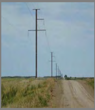
138kV Single-Circuit Single Pole Structure
