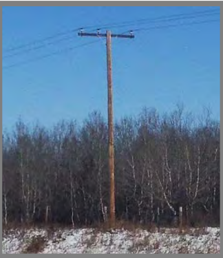
25kV Distribution Single-Circuit Structure
