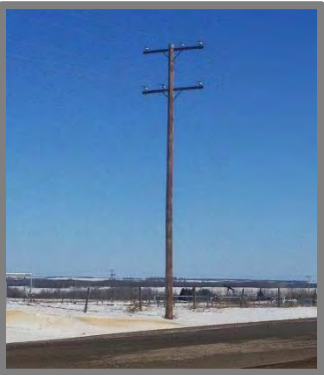
25kV Distribution Double-Circuit Structure
