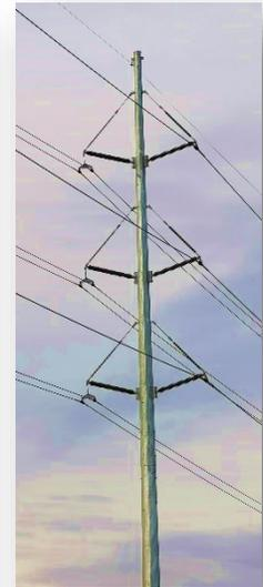
*The picture on the left shows an example of a single-circuit structure with all phases of conductor on one side of the structure.*
