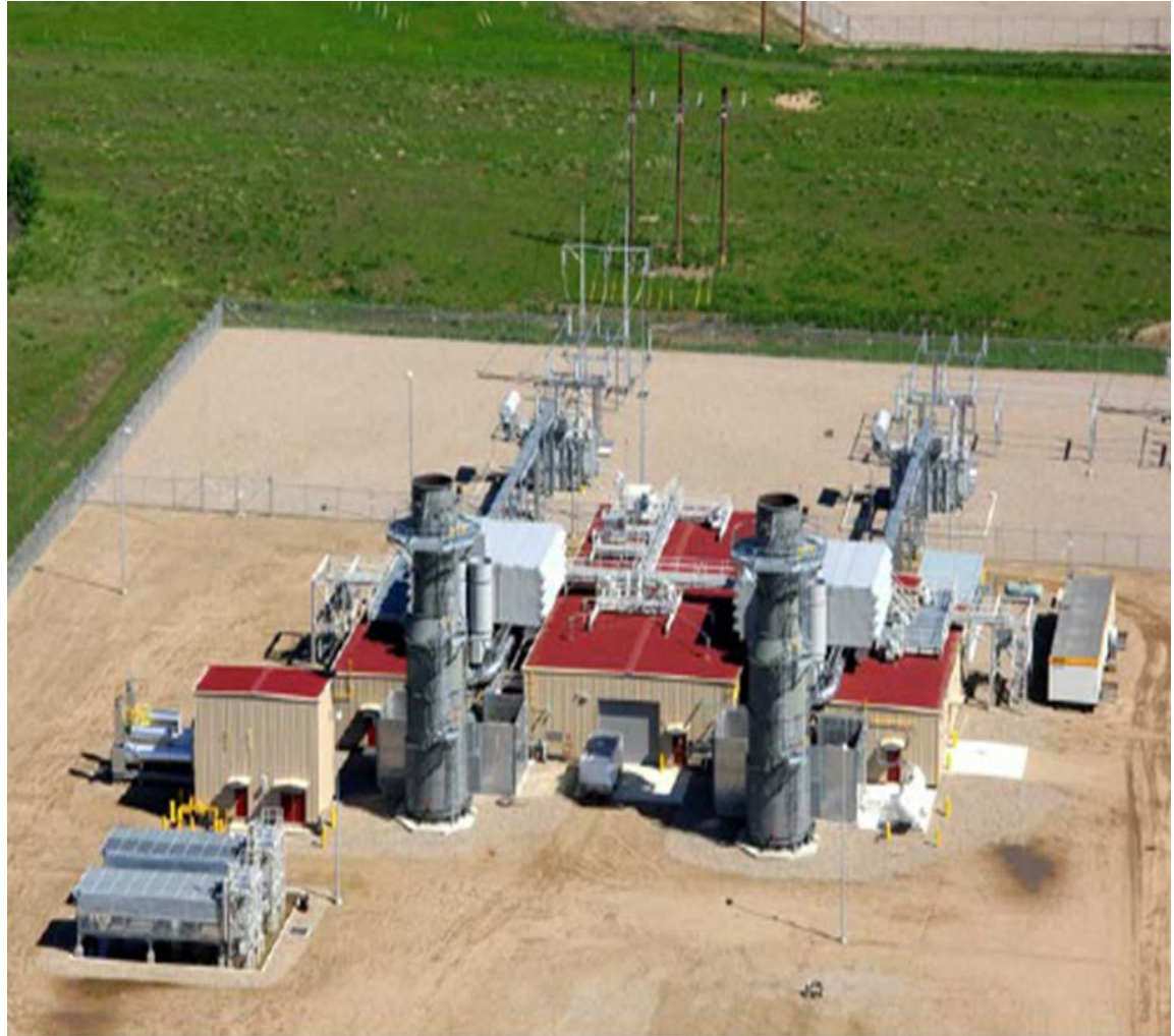
Ermine Power Station (2 x LM6000PD)
