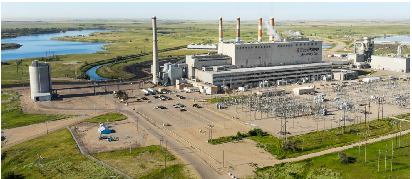
BOUNDARY DAM POWER STATION
