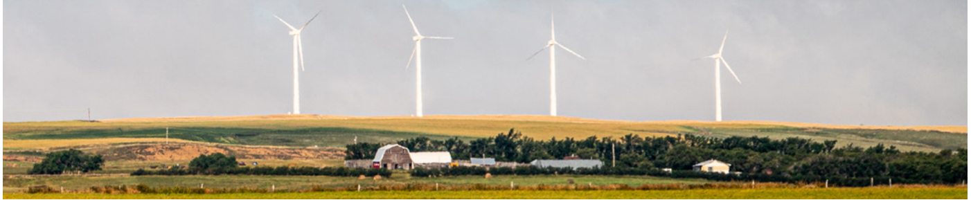
CYPRESS WIND POWER FACILITY
